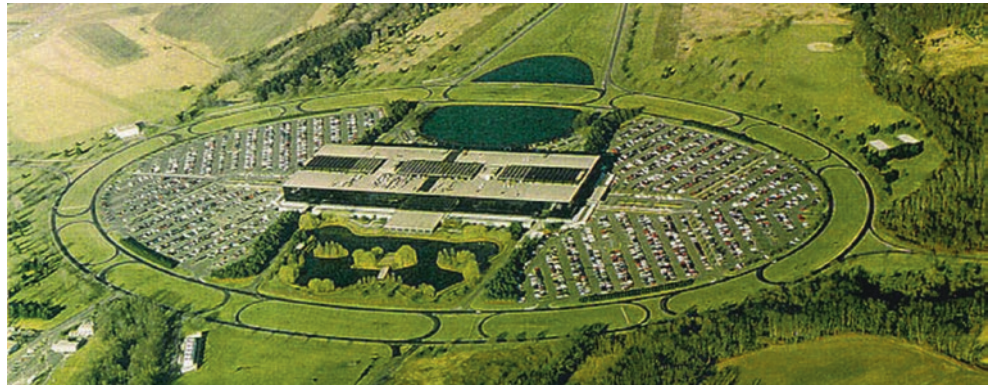
Fig. 4.1 Bell Labs R&D facility in Holmdel, NJ
